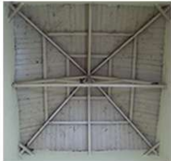
8. ROOF STRUCTURE OF STAIRWELLS
