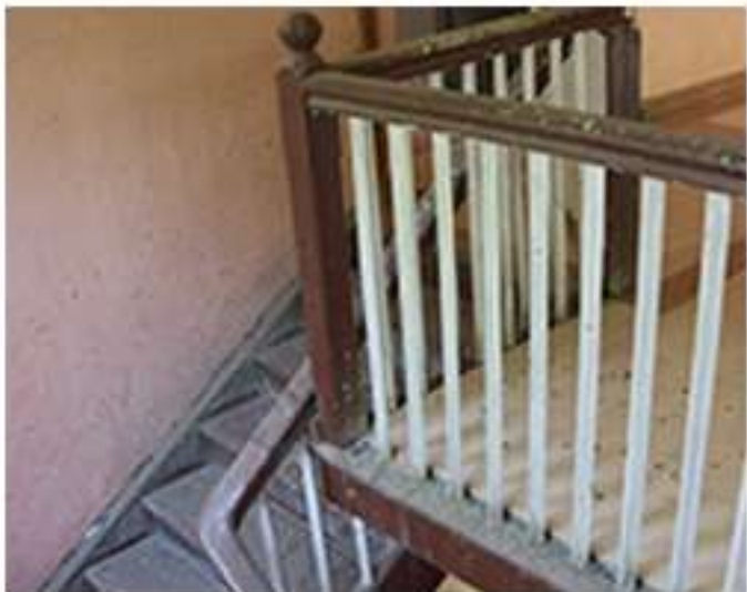
9. STAIRCASE IN THE STAIRWELLS
