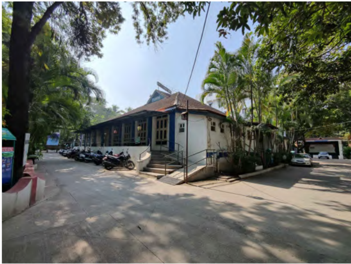
5. NORTH- EAST CORNER
