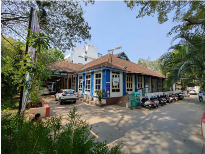
2. SOUTH- EAST CORNER
