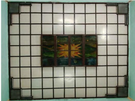
7. FALSE CEILING IN OFFICE SPACE
