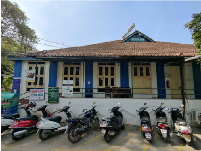
4. EAST SIDE FACADE
