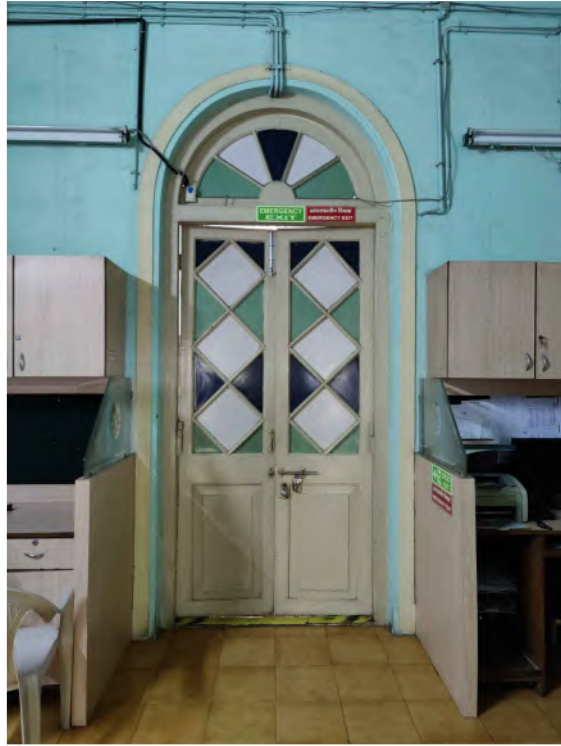
4. DOOR (D3) IN OFFICE SPACE
