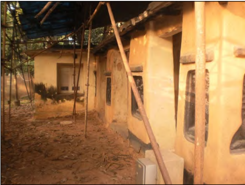
4. Exterior View of West Elevation
