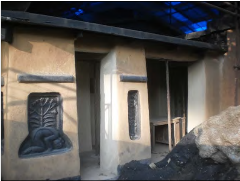
3. Exterior View of South Elevation
