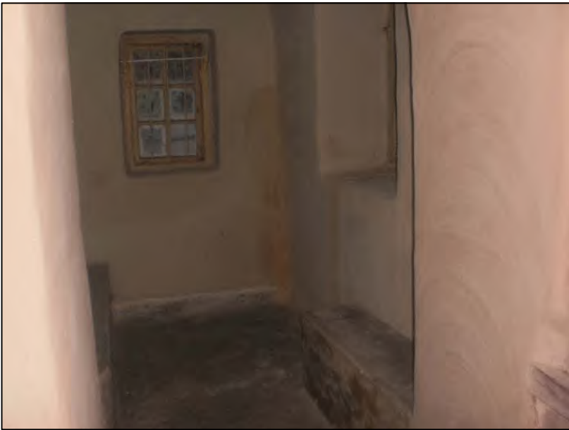
4. Interior View of Bath
