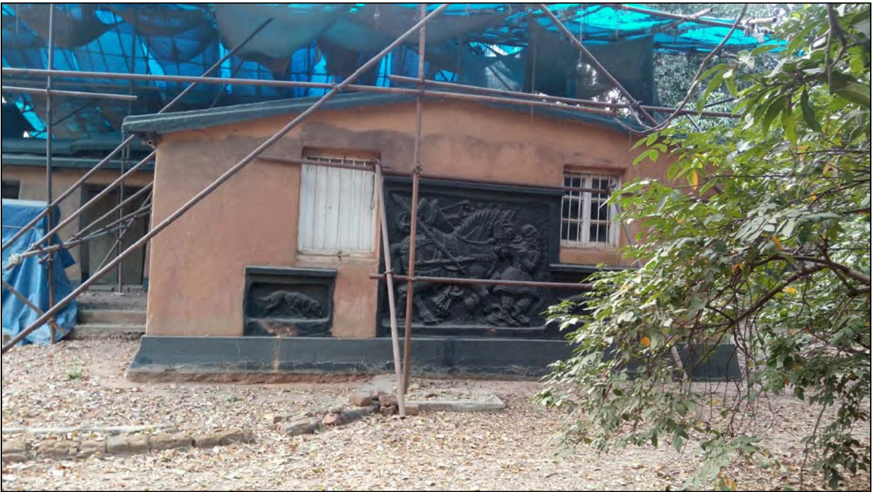
7. Exterior View of East Elevation
