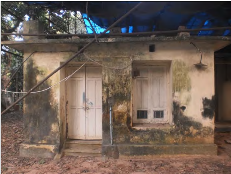
5. Exterior View of West Elevation
