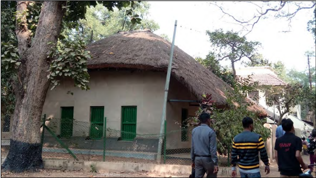
3. Exterior View of West Elevation
