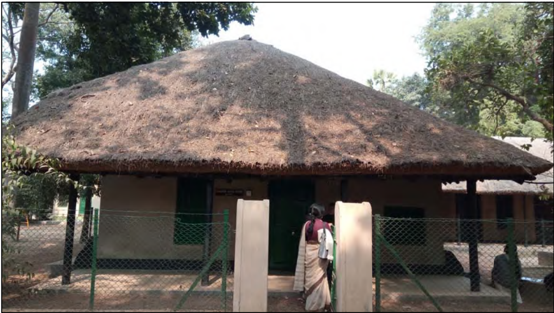
1. Exterior View of South Elevation
