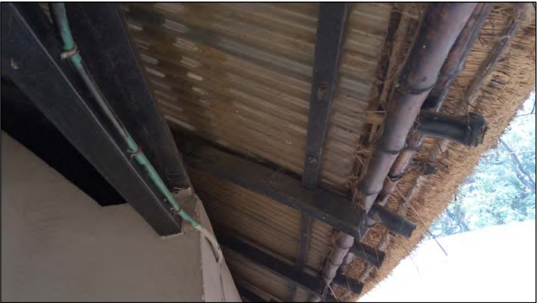
4. Details of Roof Projection
