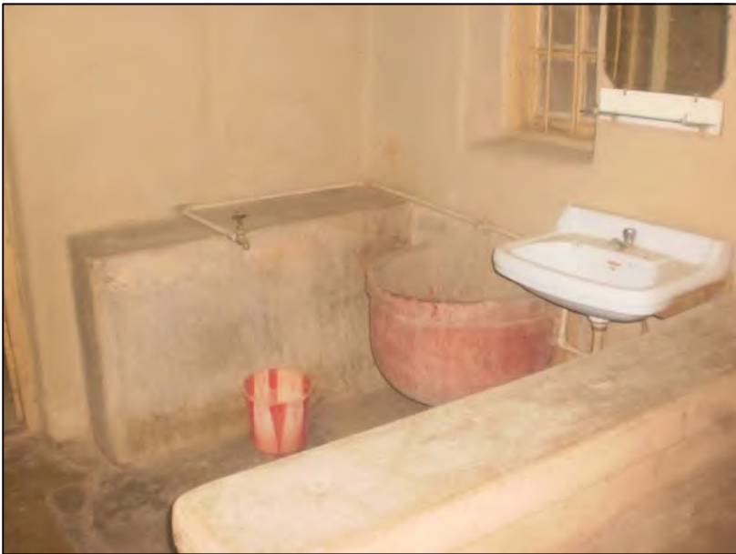
5. Interior View of Bath
