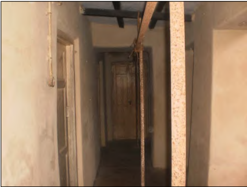
3. Interior View of East Corridor
