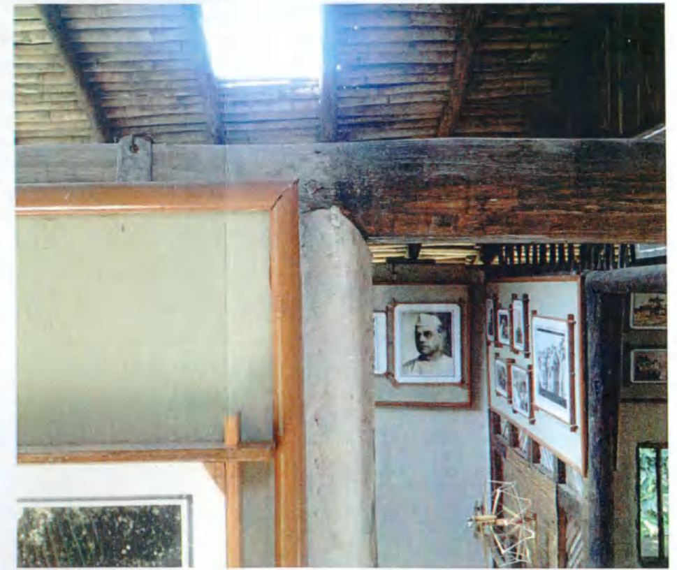
7. DETAIL OF TIE BEAM AND SEPARATION WALL
