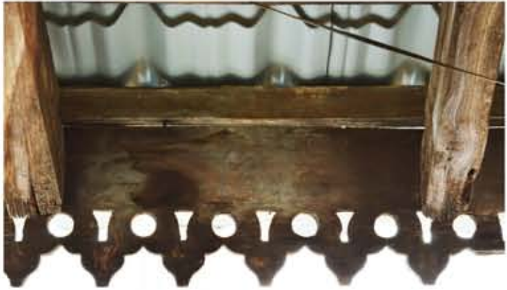
9. ROOF DETAIL (EAVES BOARD)
