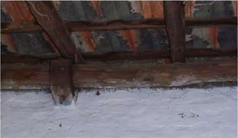
6. WOODEN BRACKET SUPPORTING THE WALL PLATE
