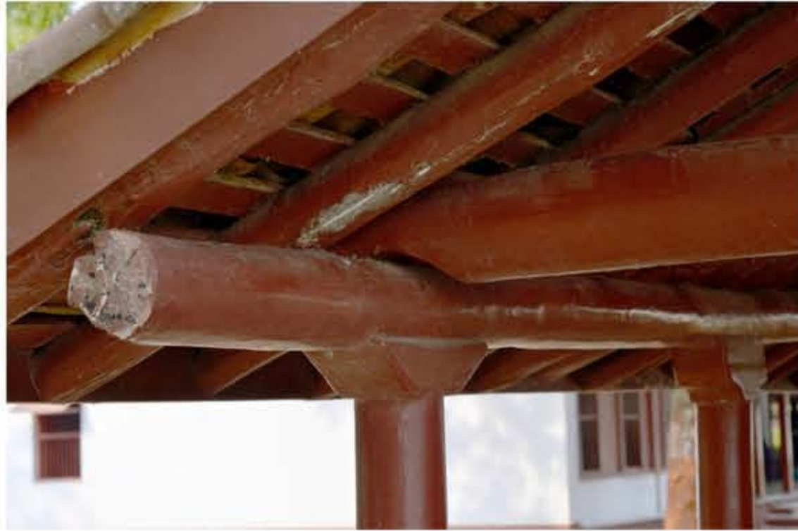
5. TRUSS AND POST JOINERY
