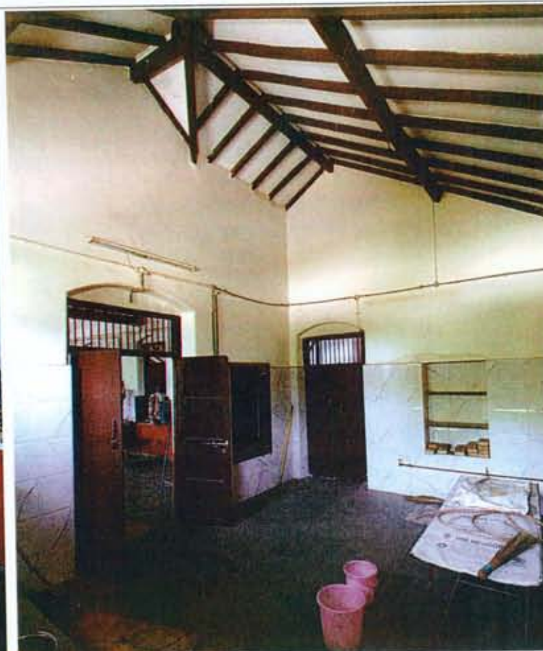
2. INTERIOR VIEW OF VAULT
