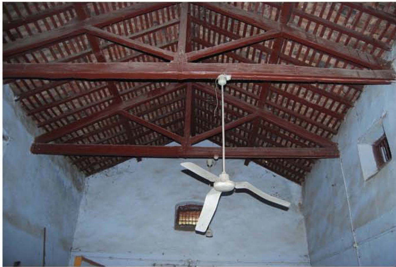
IMAGE:5 (ON LEFT) CENTRAL HALL WITH KING POST TRUSS ROOF AND ITS DETAILS.
