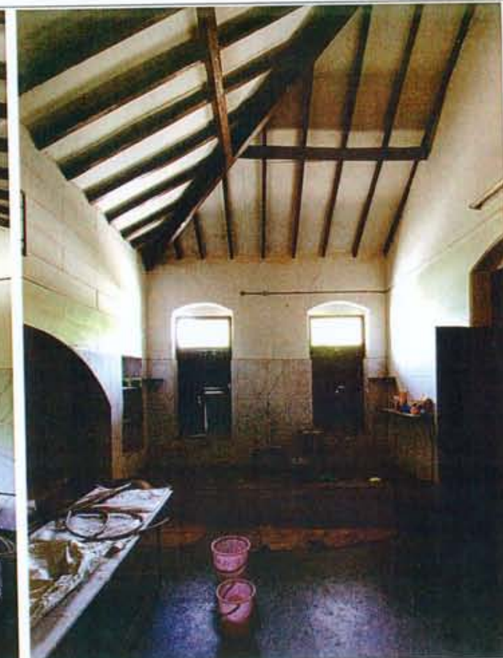
3. VIEW OF WASH AREA
