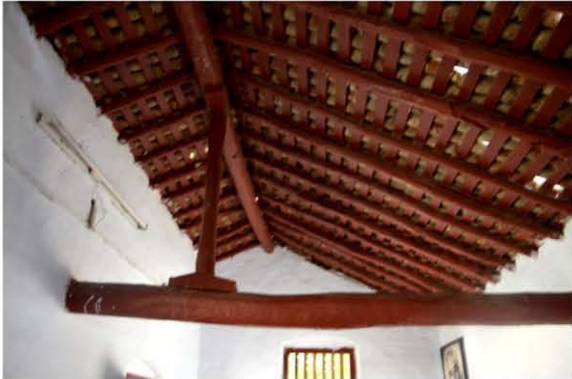
6. TRUSS AND RIDGE MEMBER JOINERY
