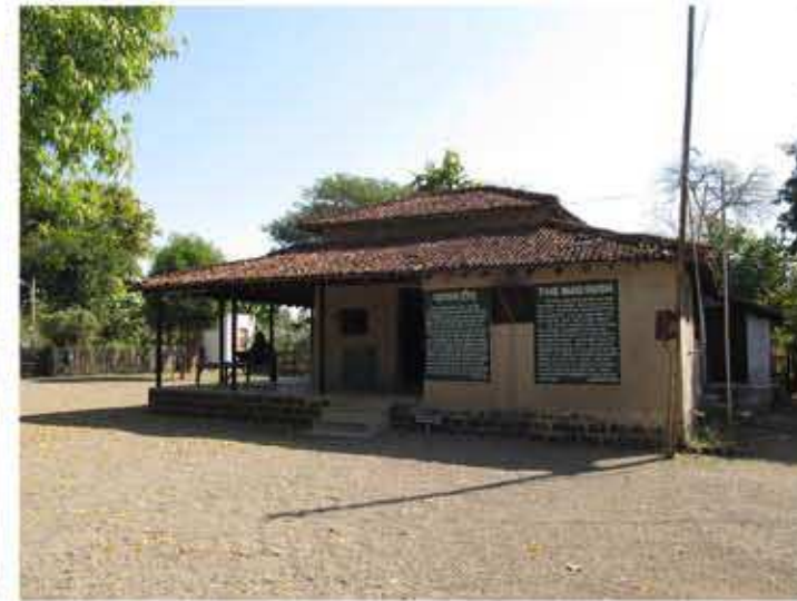
5. VIEW OF THE NORTHERN VERANDAH
