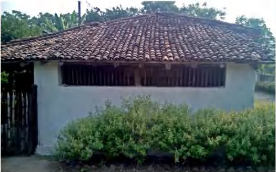
7. NORTH FACADE OF KITCHEN
