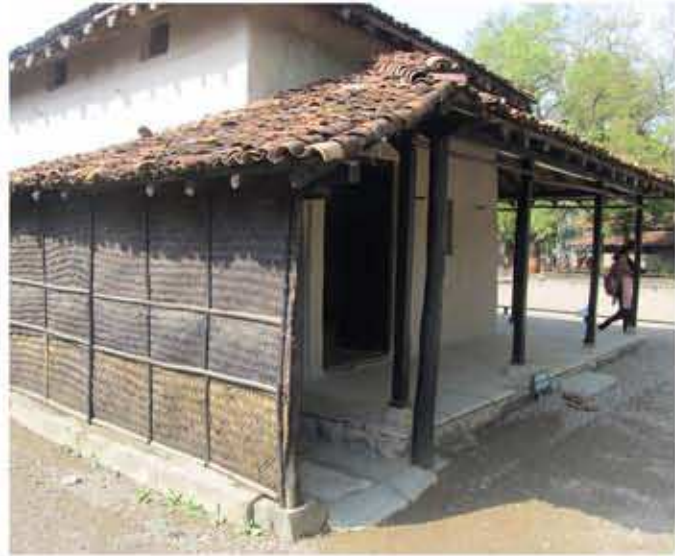
6. NORTH EAST FACADE
