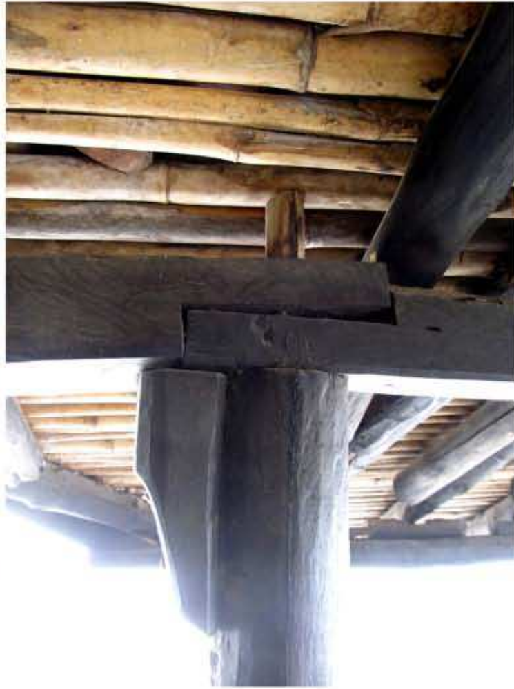
2. BEAM EXTENTION WITH POST SUPPORT
