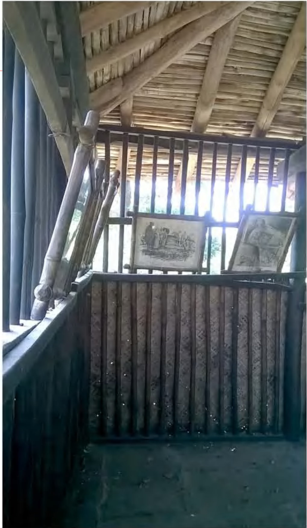
WALL COMPOSITION AND HIP RAFTER JOINERY
