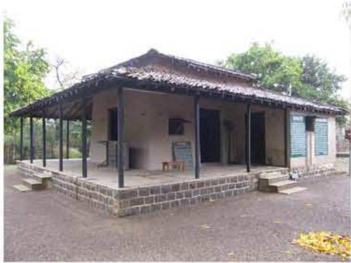
3. VIEW OF THE NORTHERN VERANDAH
