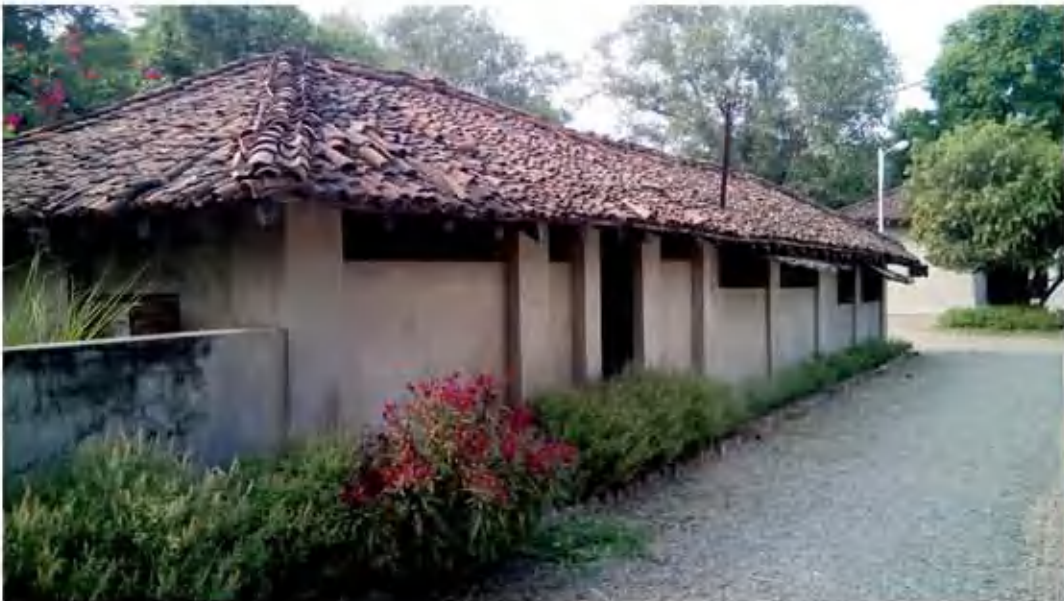
5. SOUTH-EAST VIEW OF BHOJANALAYA
