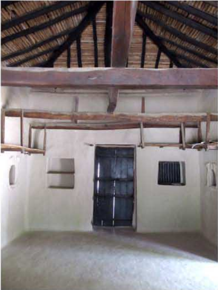
2. INTERNAL SPACE WITH WOODEN LOFTS
