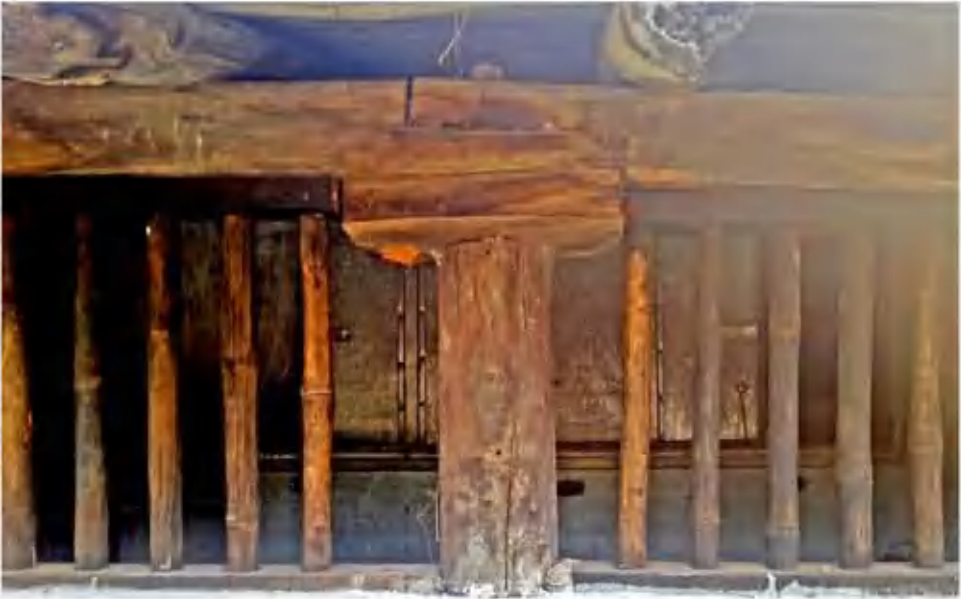
2. POST AND TIE BEAM JOINERY
