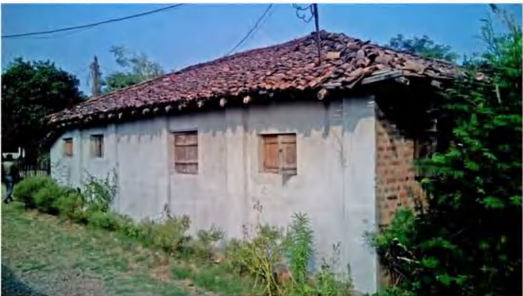
6. SOUTH-WEST VIEW OF KITCHEN
