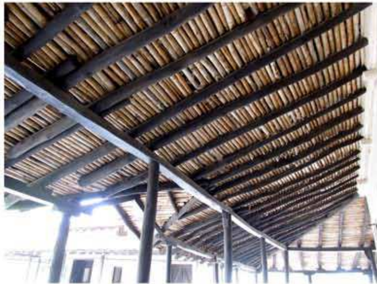
4. RAFTERS WITH MACHAAN RESTING ON BEAM AND POST
