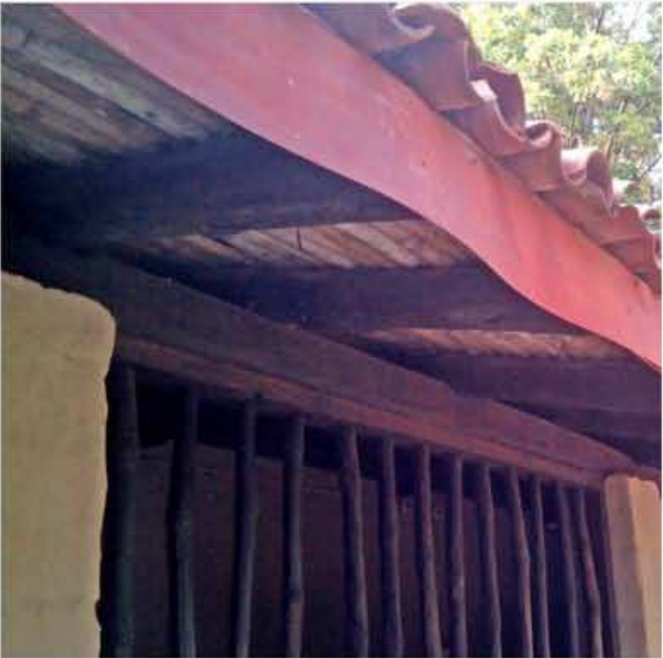
2. RAFTER AND FACIA BOARD JOINERY
