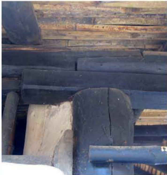
5. EXTENSION OF BEAM ON POST
