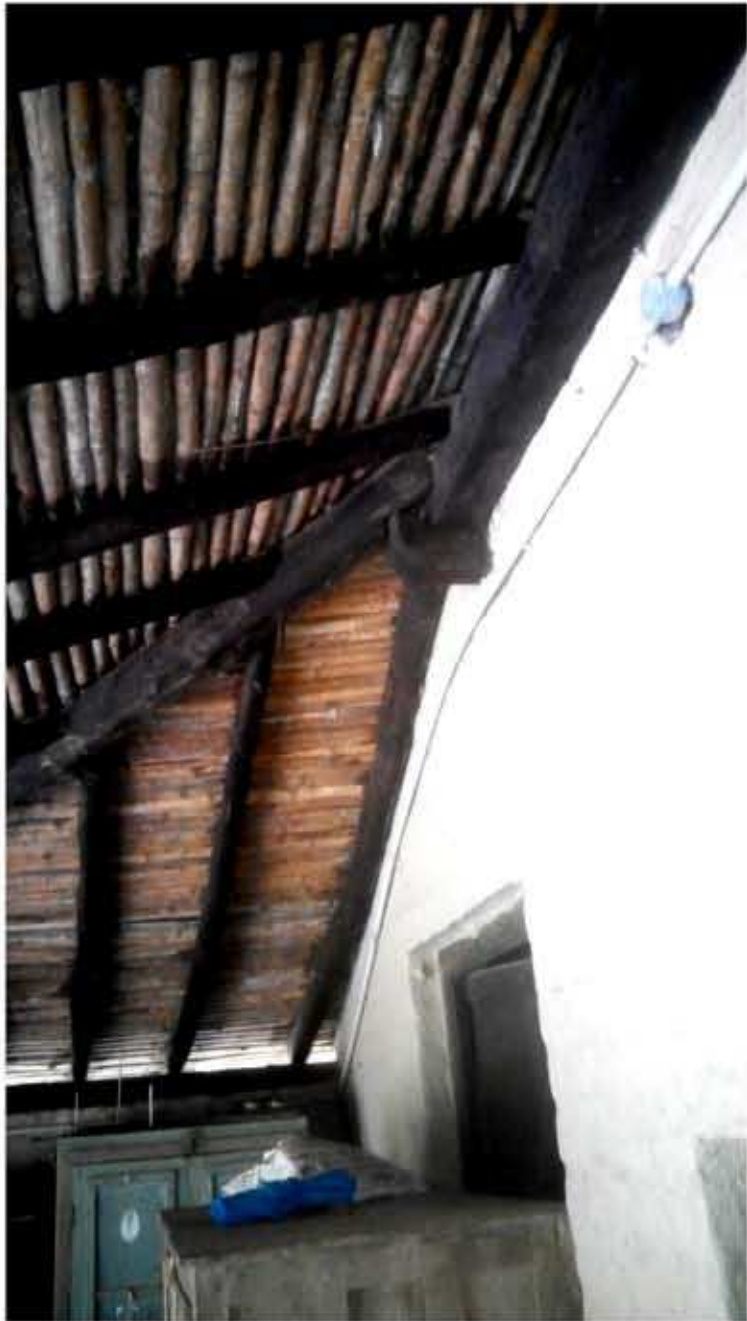
1. RIDGE MEMBER AND TIE BEAM JOINERY
