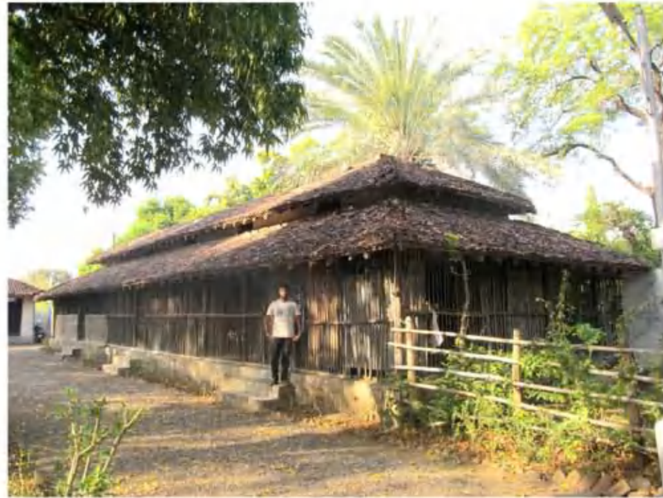
2. VIEWING THE EASTERN CORNER / VERANDAH COVERED WITH BAMBOO SCREENS
