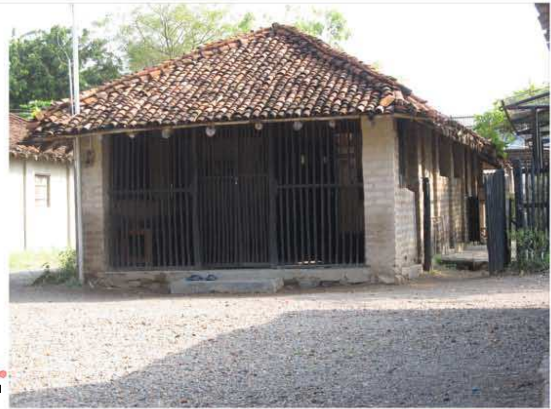
1. BHOJANALAYA BUILDING FRONT ACCESS FROM MAIN ASHRAM COMPLEX
