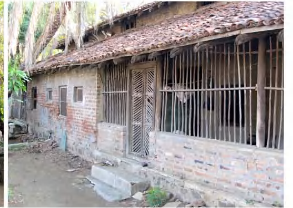
4. BAMBOO SCREENS ON BRICK PARAPET AT WESTERN FACADE
