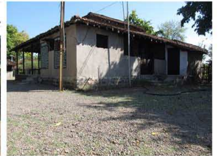
6. VIEW OF THE NORTHERN VERANDAH
