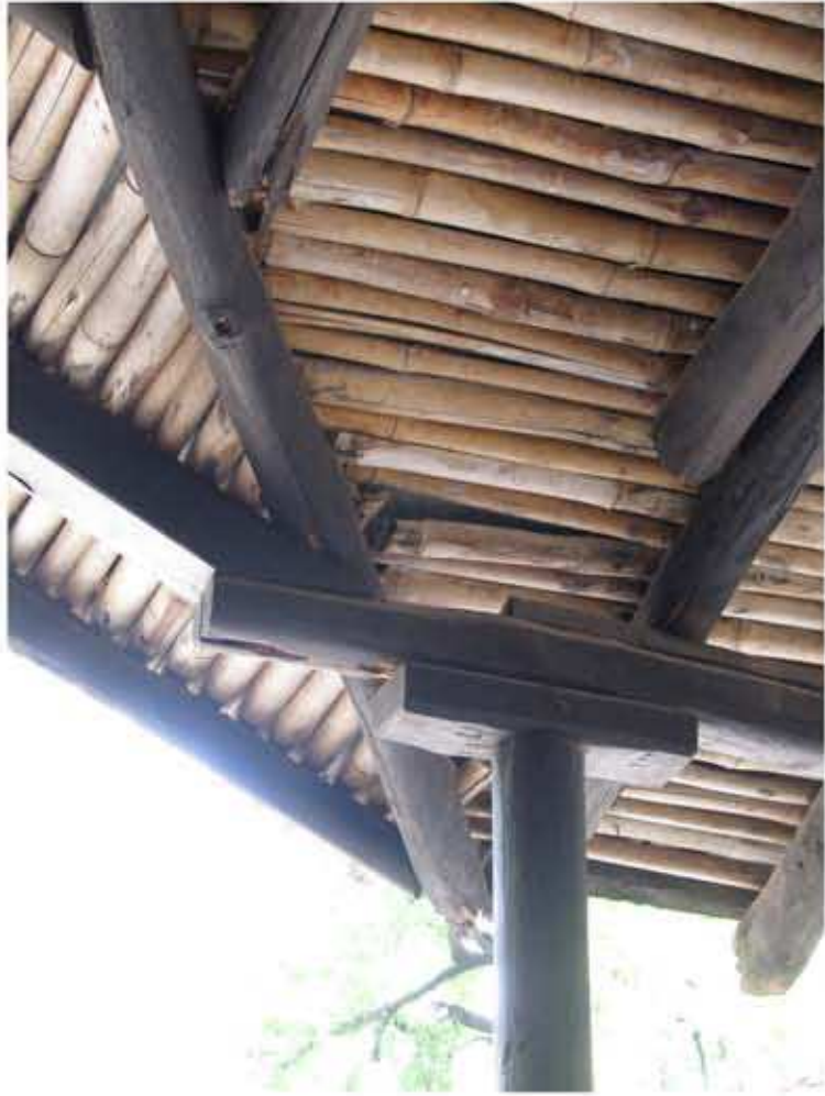
1. HIP, RAFTER, BEAM AND POST JOINERY
