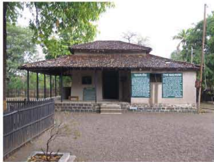
4. VIEW OF THE NORTHERN VERANDAH
